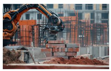
The repetitive construction work, such as brick laying and the like, can be handled by autonomous construction equipment that can get their instructions from the BIM model, or at least the contractor's version of it (liability issues have to be considered here). Having AI monitoring site safety with image recognition of video data has the capability of identifying unsafe work practices and can lead to better training for site staff.
